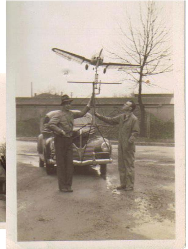
*Mallard model in skeleton form and covered and attached to a fixture mounted to an automobile as an "open range" wind tunnel.*
